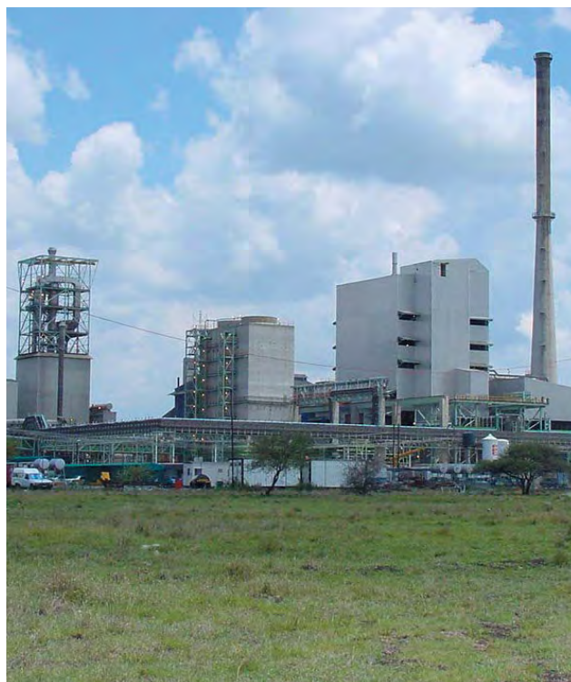
Smelter complex, Western Platinum Mine. © Lonmin.
