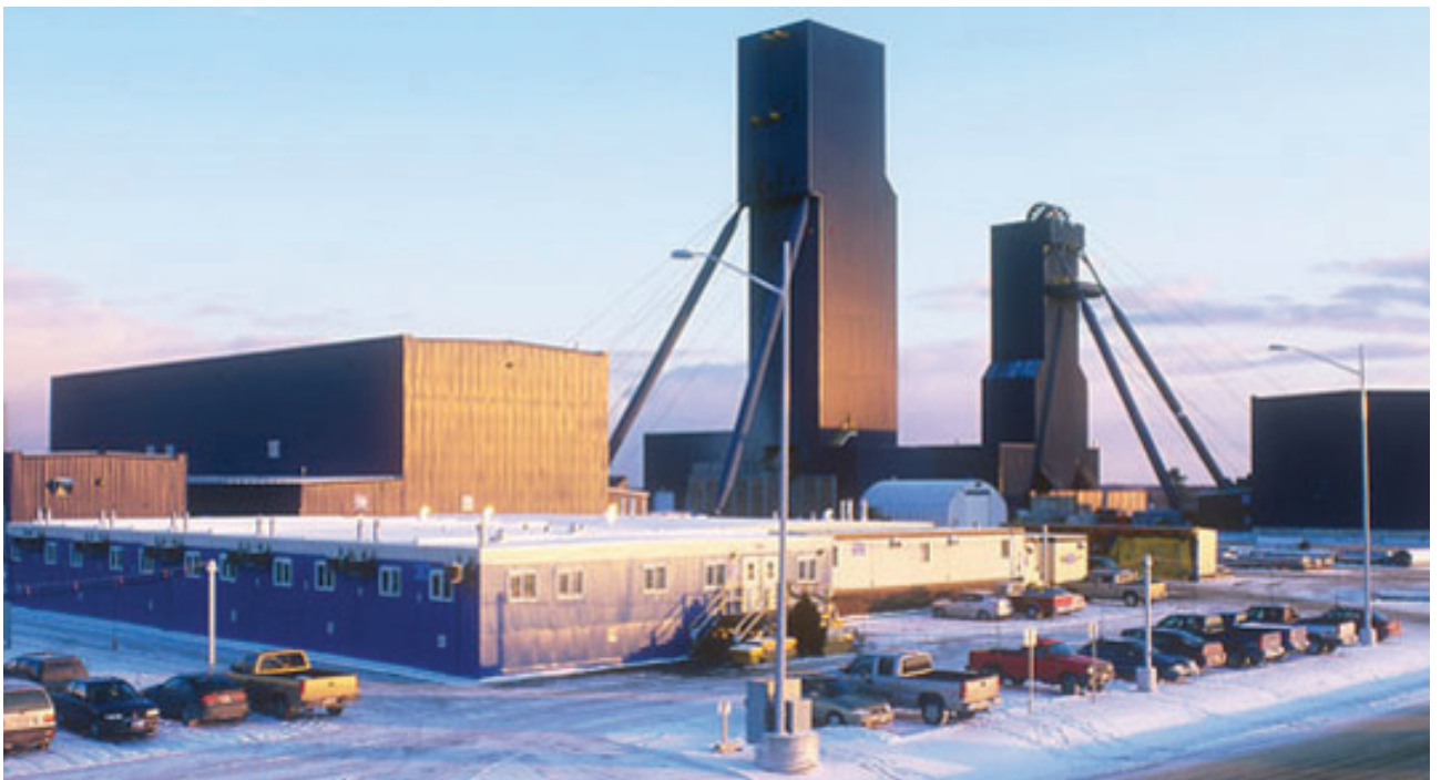
Construction of the new Nickel Rim South project in Sudbury, Canada. Courtesy of Xstrata Plc.
