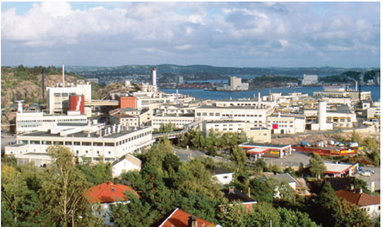
View of the Nikkelverk refinery, Norway. Courtesy of Xstrata plc.
